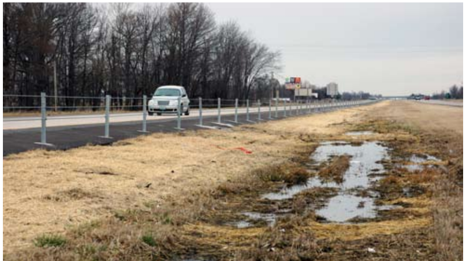
Completed I-55 guard cable system
