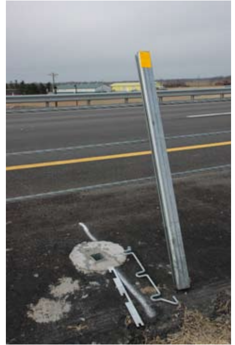
Complete guard cable structure
